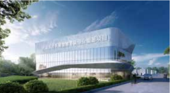
Energy Storage Project in Pinghu, Jiaxing City
